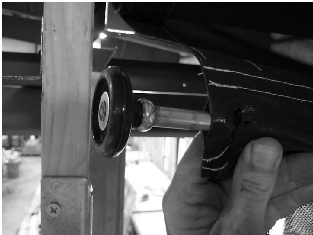
Photo #14 (Roller Installation)
