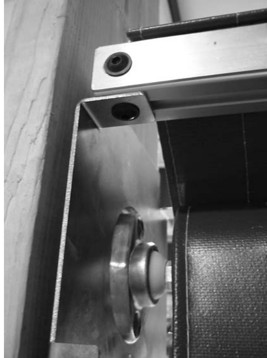
Photo #12 (Double Baffle Installation)
