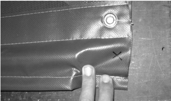
Photo #5 (Top of Stiffener Tube)
