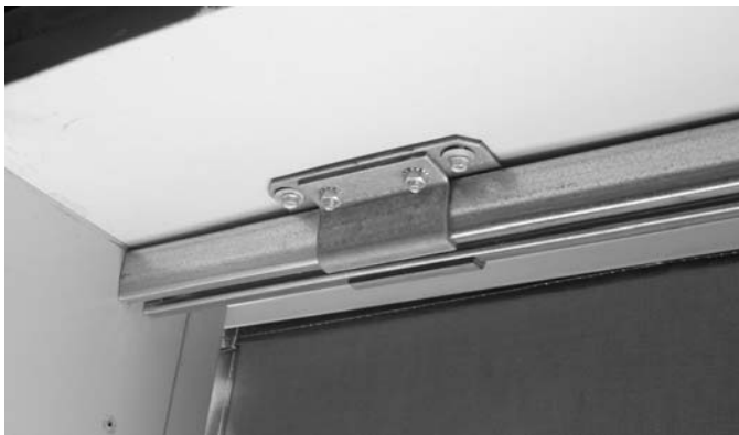
Photo #1 (Track and Splice Mounting)
