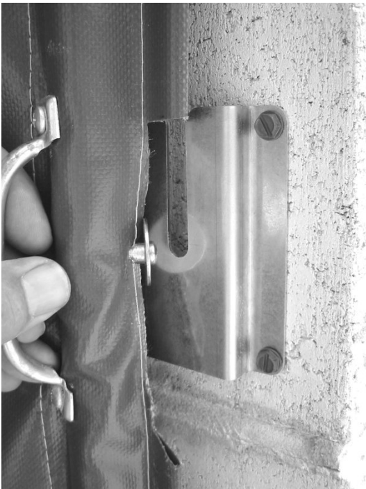
Photo #7 (Slot Lock Bracket Mounting)
